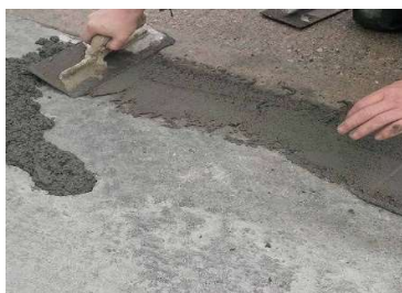
Repair of surface imperfections using cementitious repair mortar
