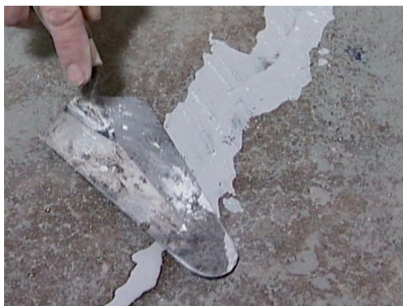
Repair of cracks using Flexseal PU245 or PU440
